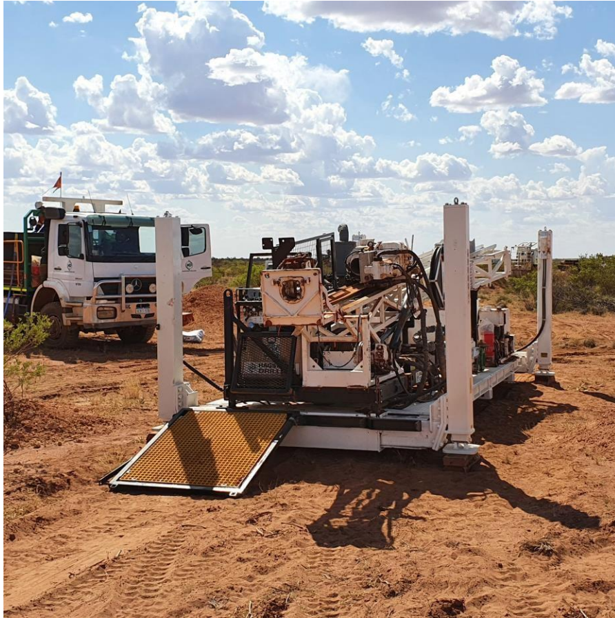
Lightweight drill rig to assist mobility
